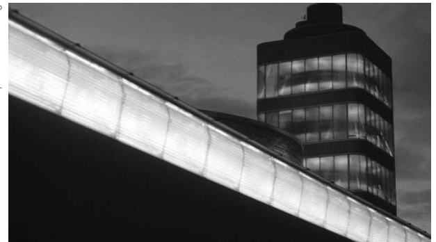
S.C. JOHNSON &amp; SON, INC. RESEARCH TOWER
